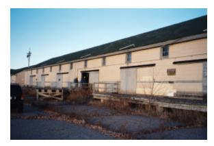
Building 1885-2 has exposed roof and walls and large dimensional lumber columns and reuses with minimal interior finishes and concrete slab and stem walls.
