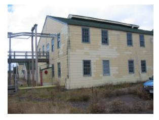
This building had water damage, high degree of entanglement of MEP systems and all wood surfaces were painted, assumed to be lead-based paint.
