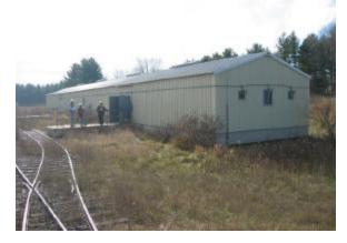
Building 1750-26 is a metal frame and cladding on concrete slab. Slab contains mastic may be asbestos containing material. Metal frame and exterior skin are either entirely recyclable or able to be dismantled and reassembled elsewhere
