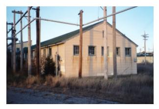
Building 30306 is framed in small dimensional lumber with ceiling and interior wall drywall and concrete slab.
