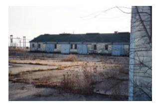
Building 305 had a light wood frame exterior, exposed roof structure, 2x sheathing and minimal interior finishes There were significant numbers of openings in the exterior walls and a concrete slab.
