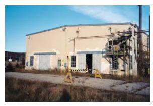
Building 700 had an exposed roof structure and walls and large dimensional lumber with minimal interior finish All wood appeared to be lead-based paint, salvage % dependent on reuse options or stripping of LBP. It had a concrete slab and concrete pits.
