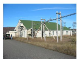
Building 224 had large sized lumber unpainted lumber trusses in the roof with concrete or CMU first-story exterior walls and a large amount of non-salvageable interior finishes.
