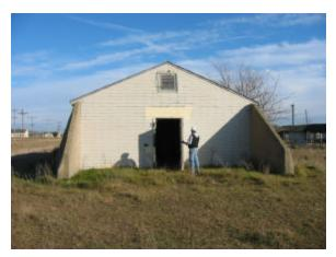
Building 6586-5 had 3 of 4 exterior walls that were poured concrete, the roof structure was salvageable, and sheathing on the one wood-framed wall was asbestos-containing materials.
