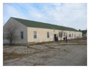
Building 6822 had an exposed roof structure with plywood sheathing with concrete slab. Exterior sheathing is granule asphalt material over suspect friable asbestos fiber board.
